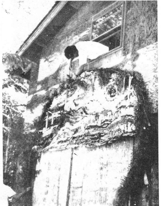
Raising the seal to the west side of the Press Building.
